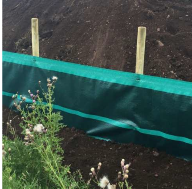
Figure 4 - Detail of Silt Trap Fence
